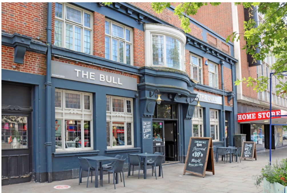
The Bull Inn façade of 1927, Market Place.
