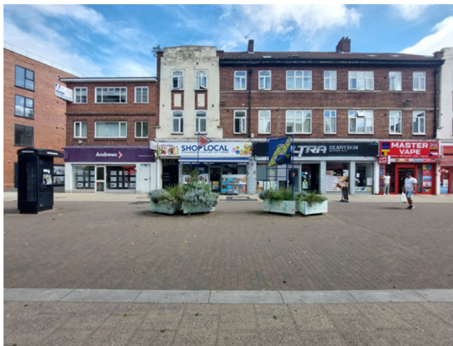
Degrading façade condition in North Street
